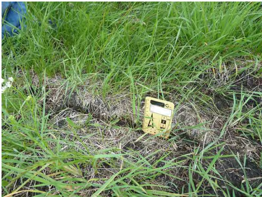
Photo 72. Ground crack with vertical displacement. 42.704152°/ 22.976076°
